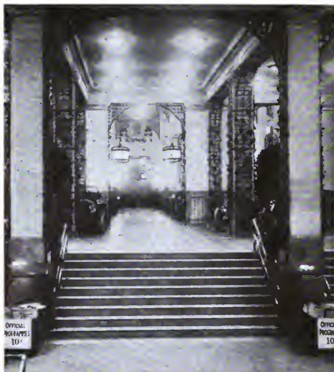
Main entrance to Grand Central Palace
